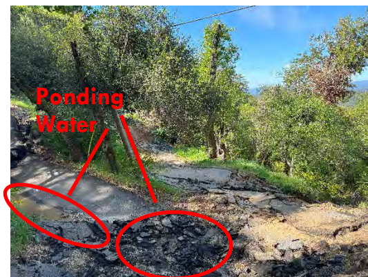
Exhibit 5 Northside of Scarp, Looking Southwest
